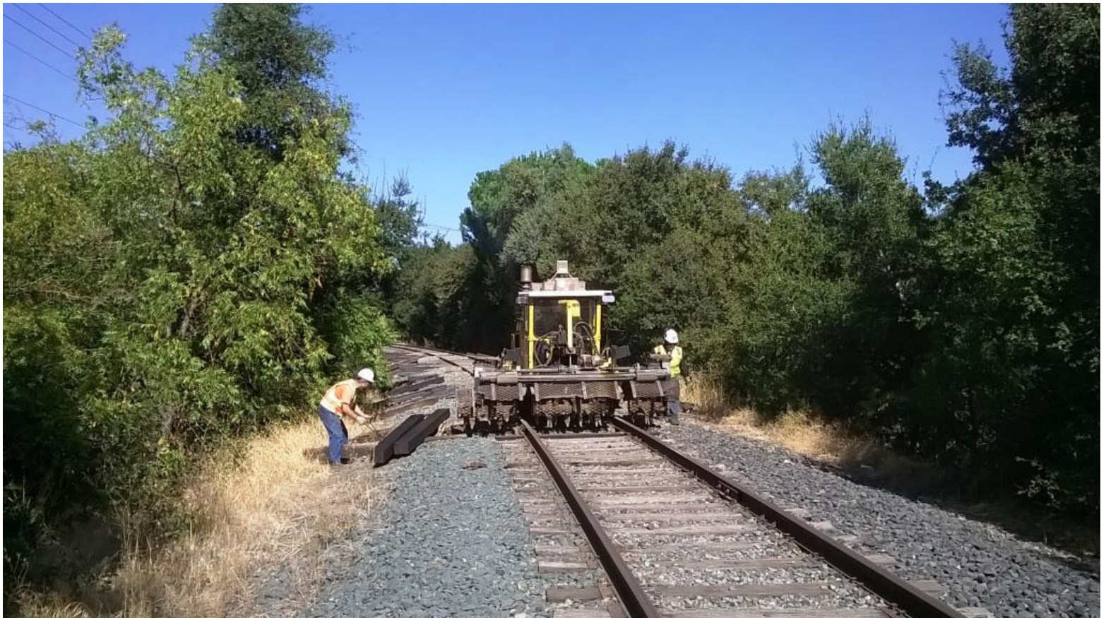
John and Joe arrange the placement of new ties
