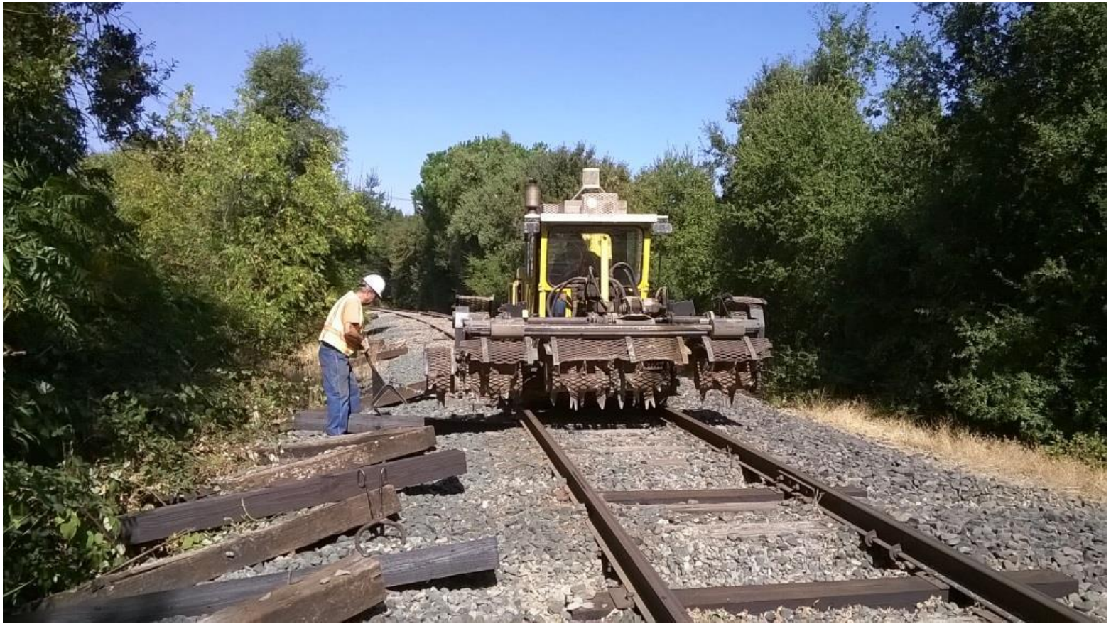
John attaches the grapple on the winch to a new tie which Mike F. in the scarifier pulls under the rails
