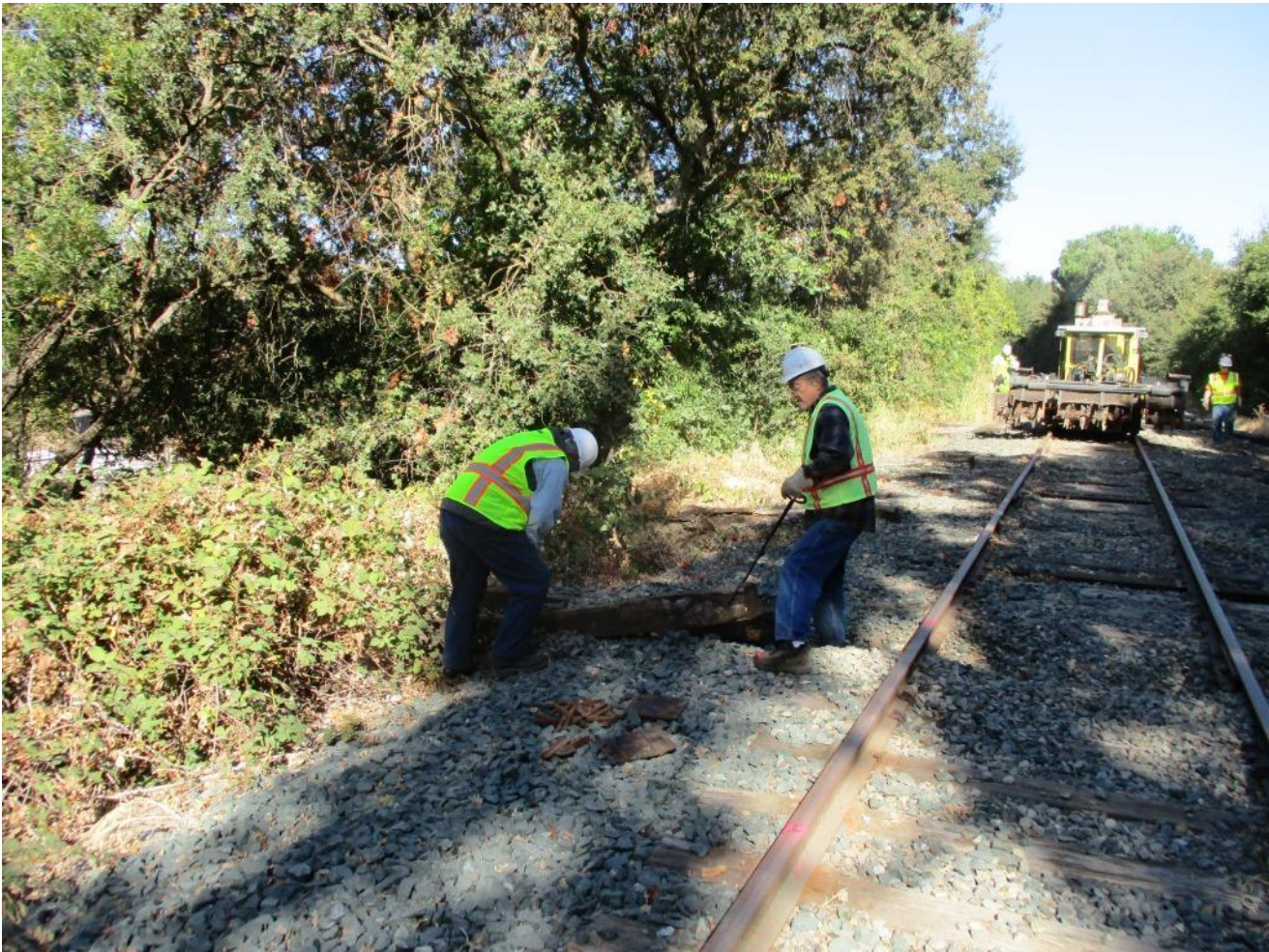
Art and John move old dead ties out of the way
