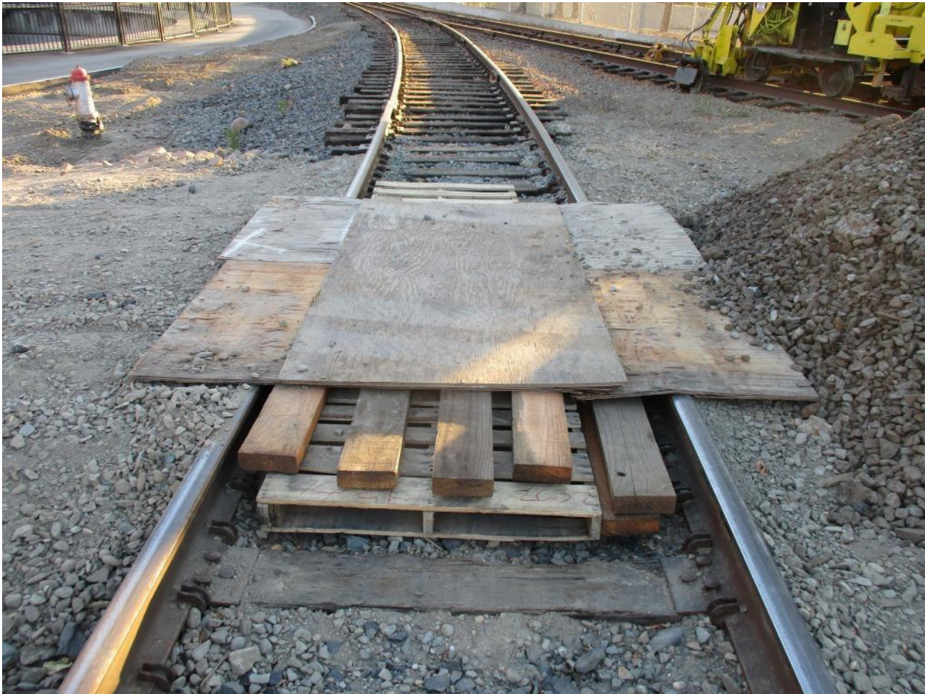
STOP! STOP! STOP! An illegal crossing built over the Interchange Track could have spelt trouble for the motorcar with two-tons of ties behind it
