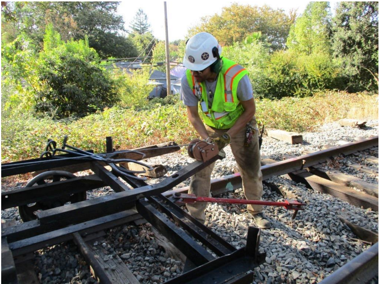
Kyle cranks on the winch and pulls the rail-lifter onto its cradle
