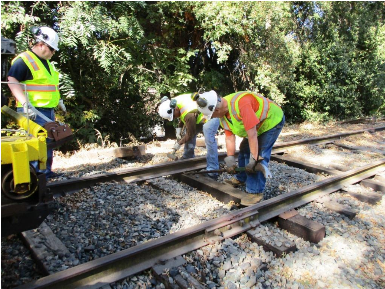
Before the rail-lifter got deployed, Dave and Clem attempt to nip-up the rail to shove a tie-place beneath
