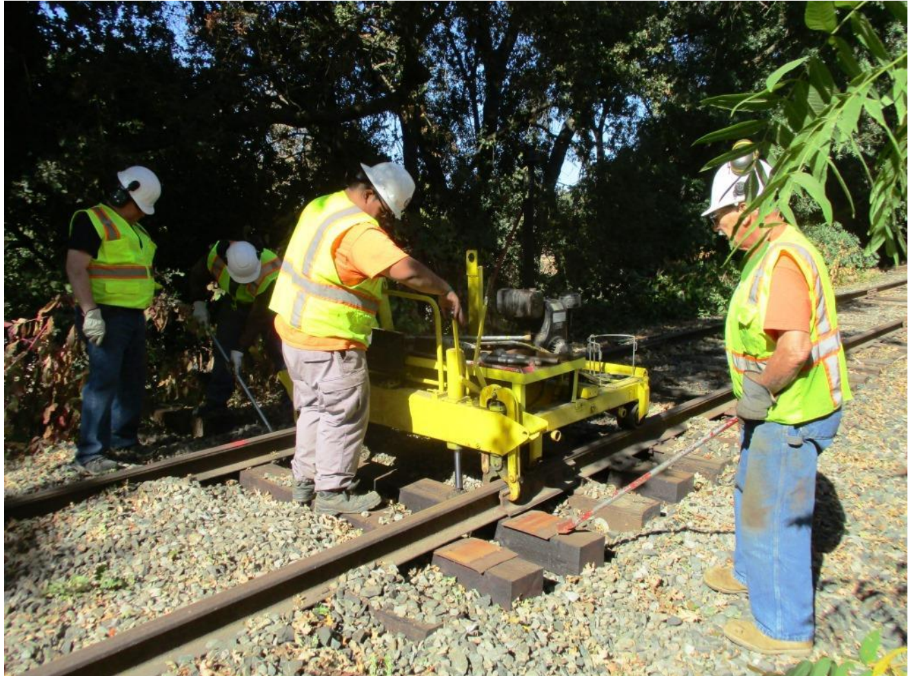
Anthony operates the rail-lifter while Dave and Clem insert new tie-plates
