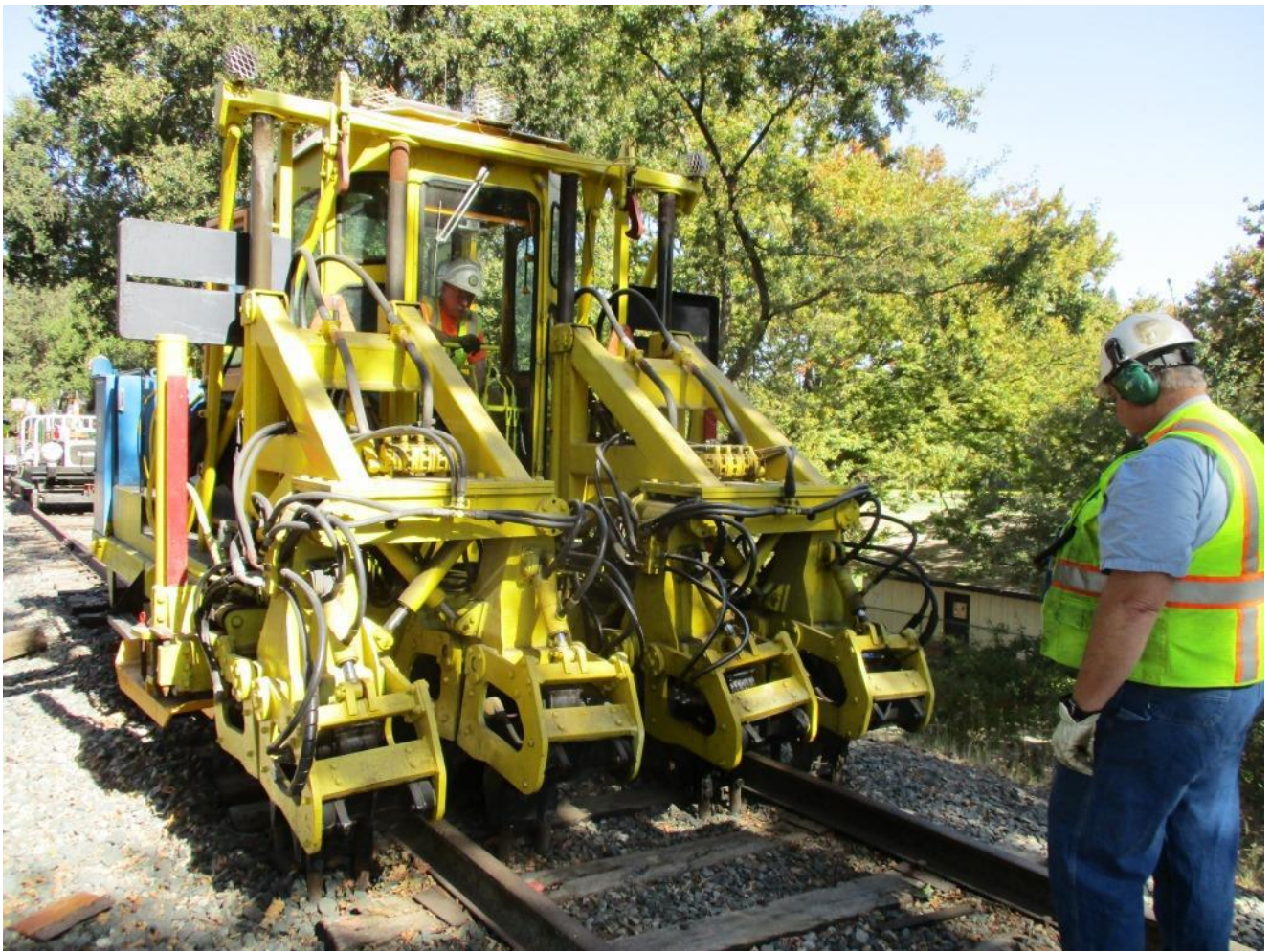
Chris C. guides Mike H. in the tamper
