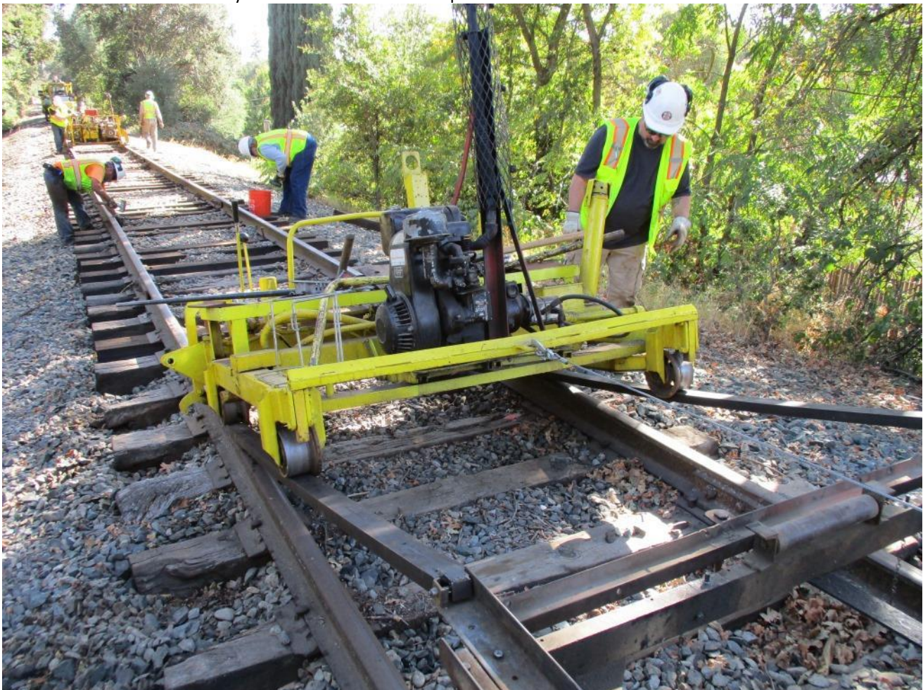
Joe and Art continue setting spikes as DJ makes sure the rail-lifter stays on the rails
