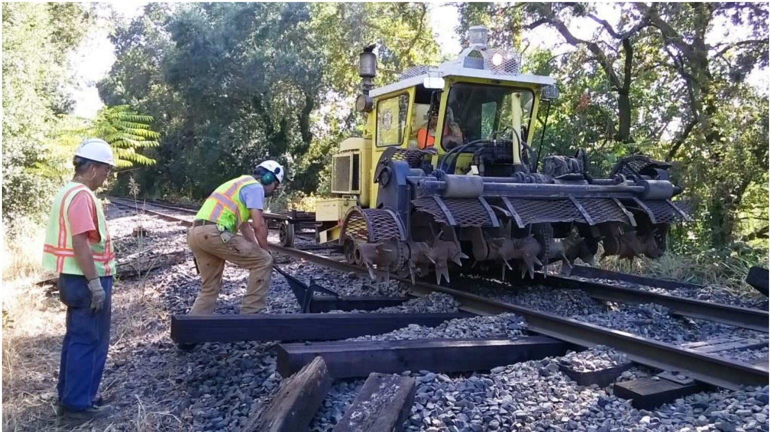
Kyle guides a new tie under the rails as Mike F. in the scarifier pulls it in
