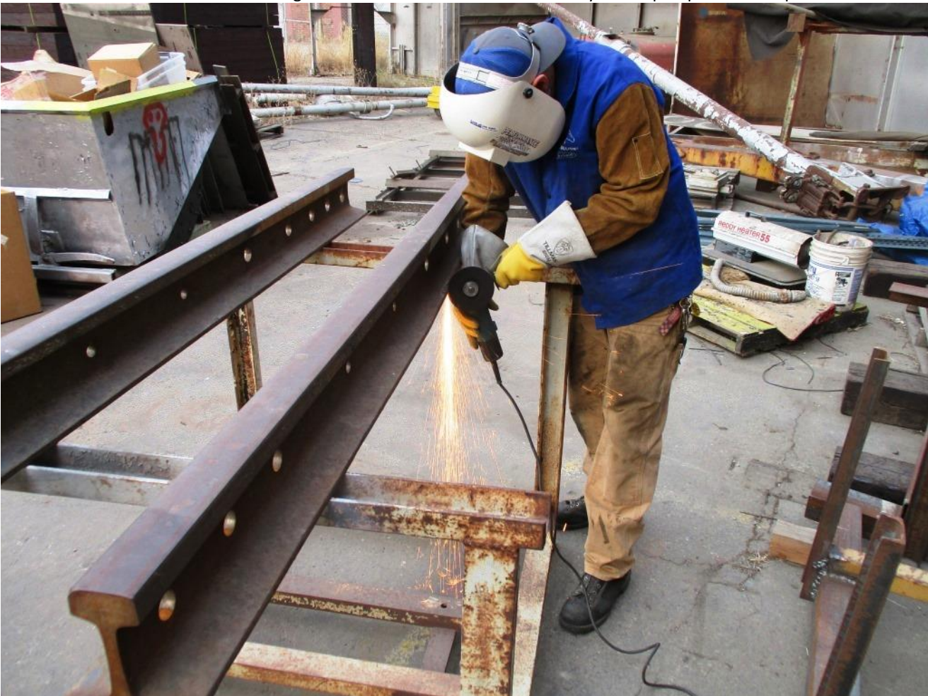
Kyle grinds-down the offending portion of the wing-rail for Switch 19
