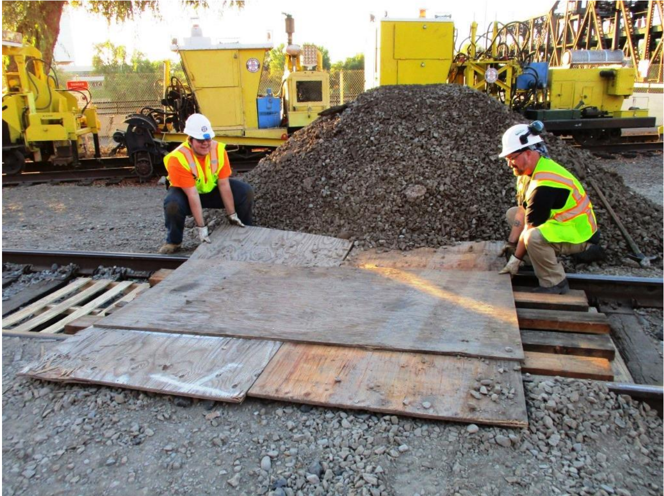
Chris and DJ dismantle the illegal crossing which was attached to the ties beneath with lag-screws
