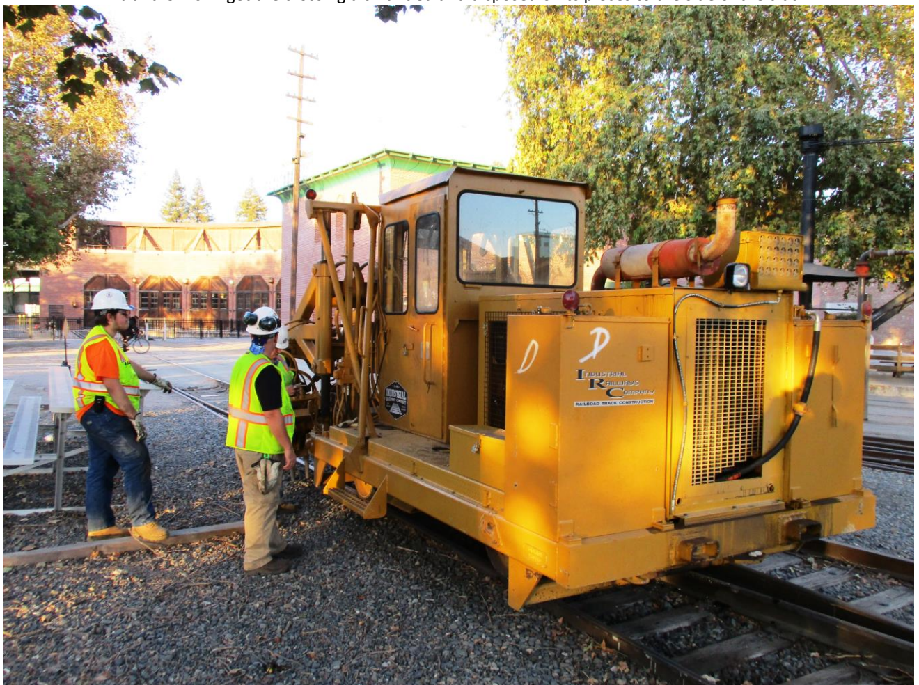
A new impediment: the contractor's tamper blocks both the South Turntable Lead and House Track thus forcing us to abandon our move
