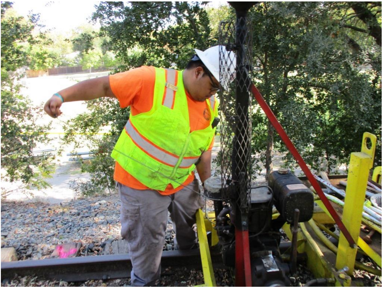
With one pull on the pull-start, Anthony brings the rail-lifter to life
