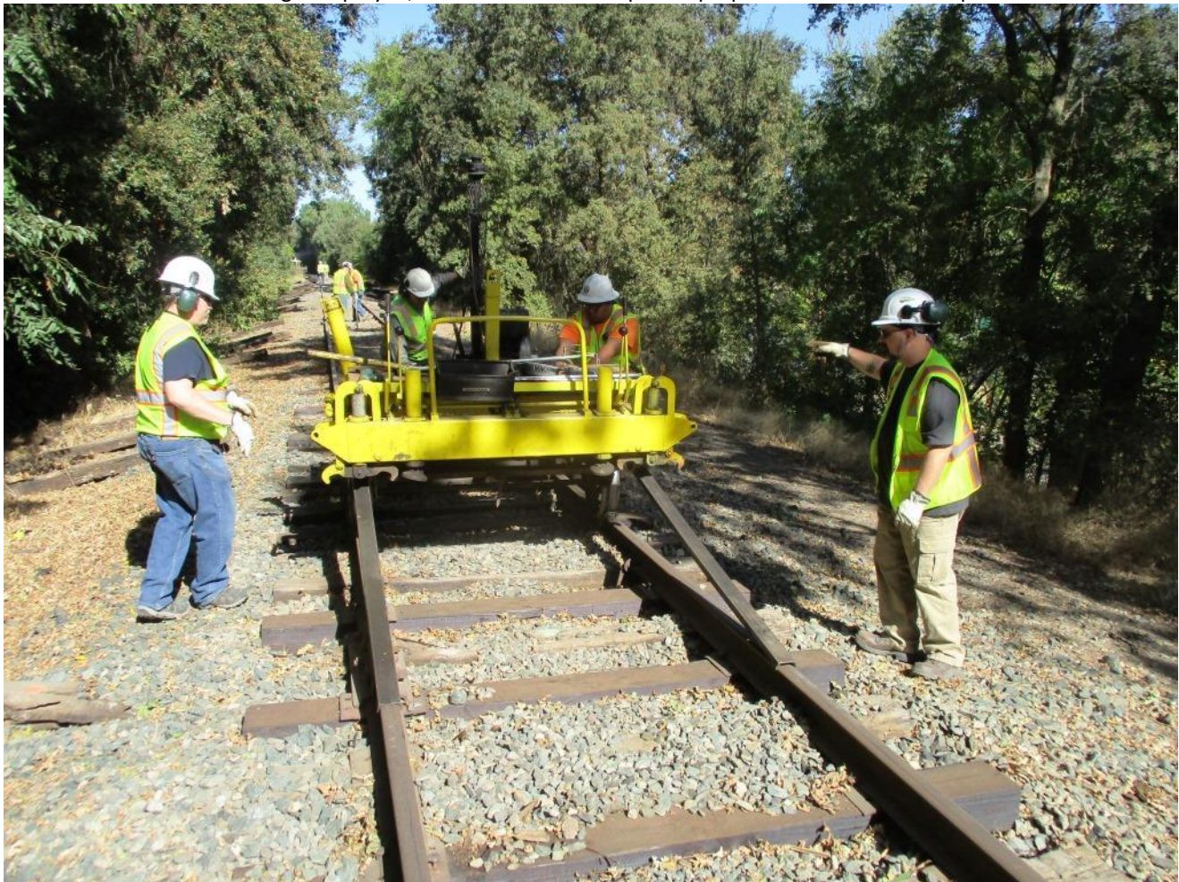
Robert, Steve, Anthony, and DJ deploy the rail-lifter
