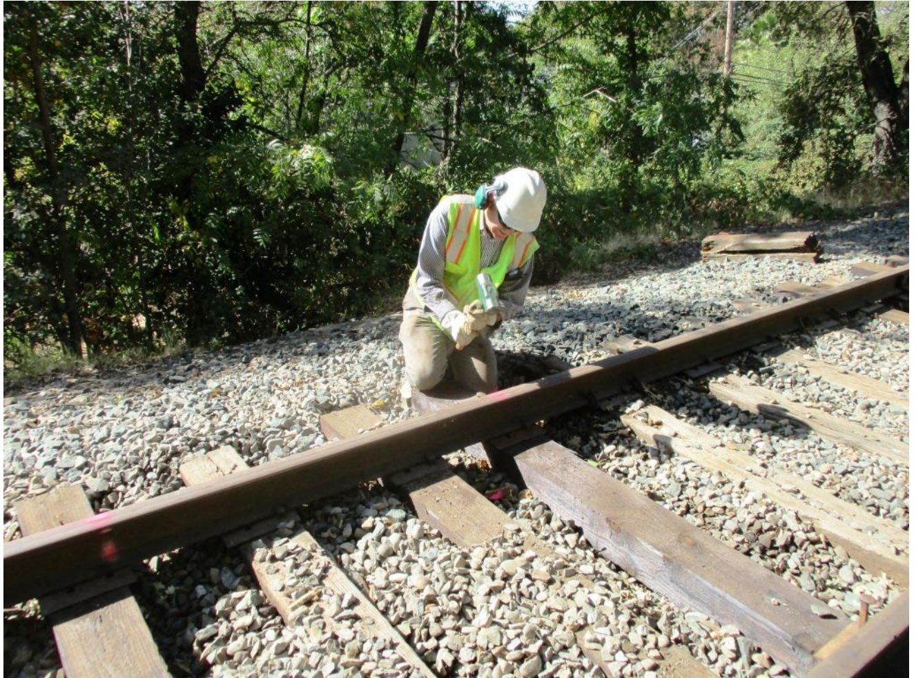
With all tie plates distributed, Steve starts setting spikes
