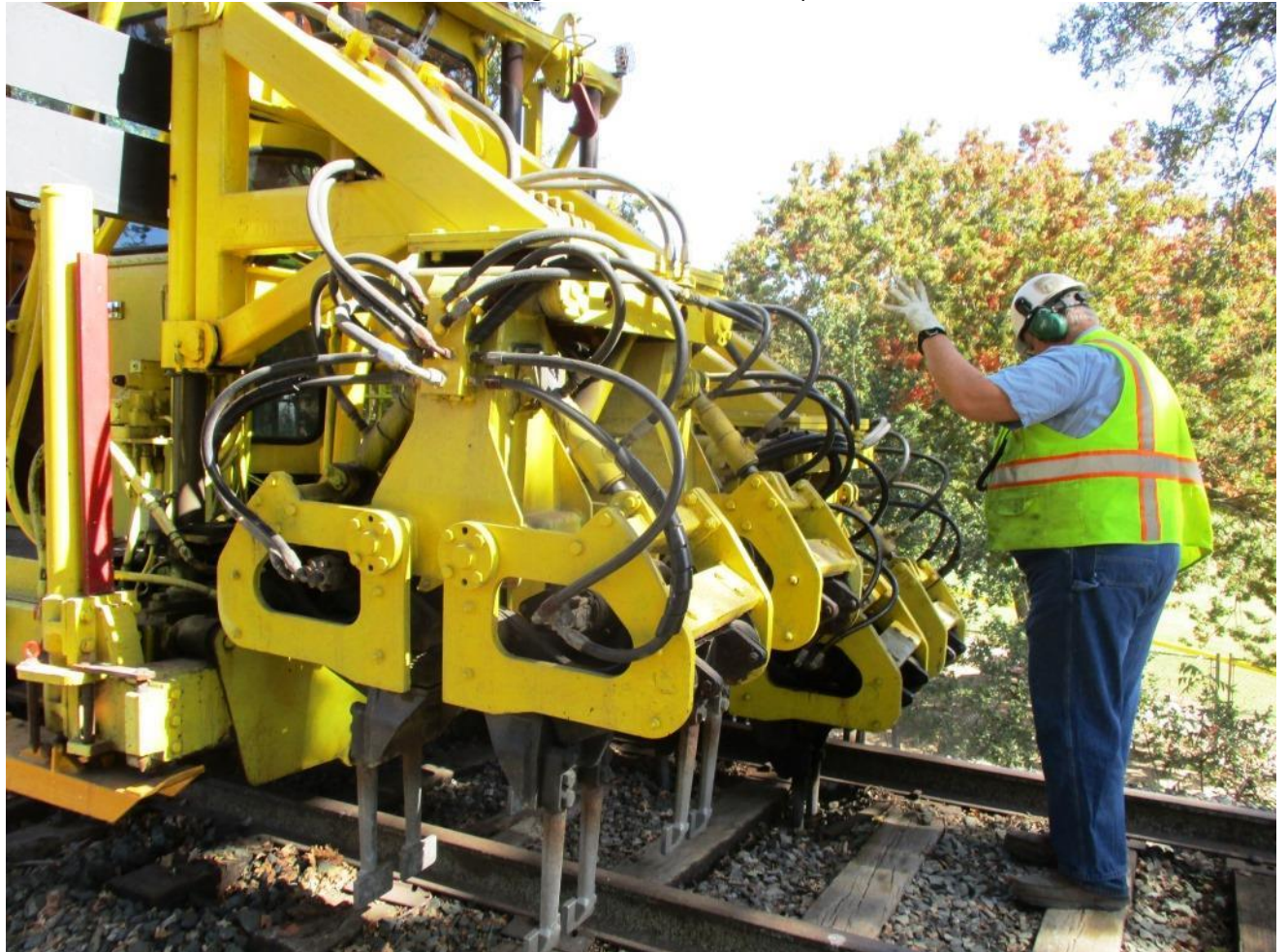
Chris C. guides Mike H. in the tamper as it is used to straighten skewed ties
