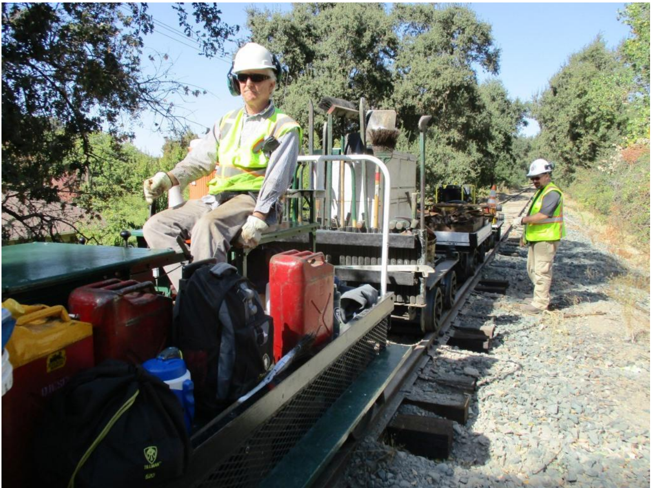
Steve and DJ distribute tie-plates down the line
