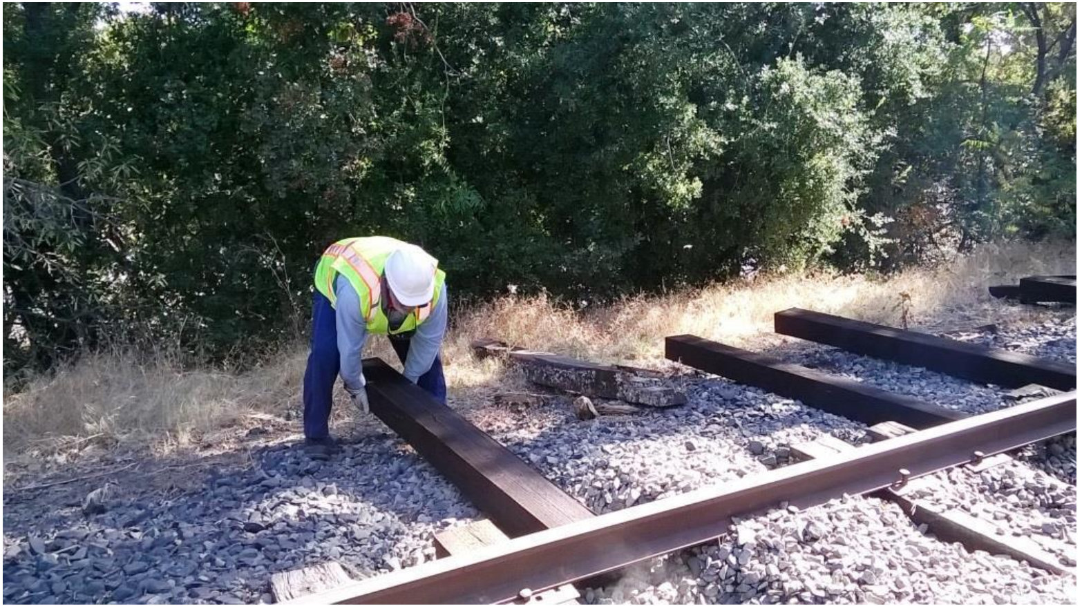
Art moves a new tie into position for insertion
