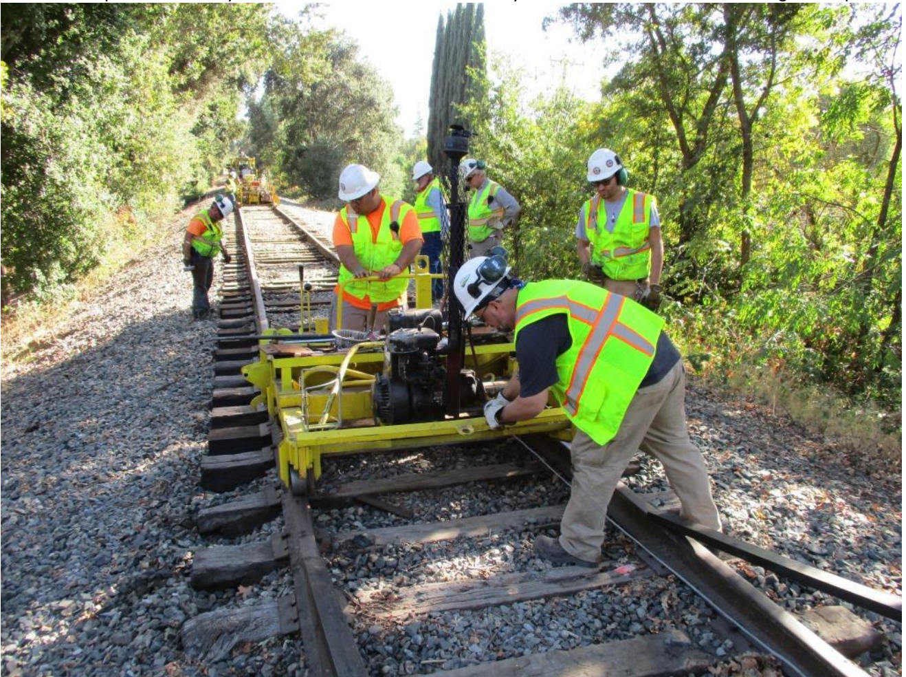
Time to put our toys away: Anthony, Kyle, and DJ get the rail-lifter ready to be stowed on its cradle
